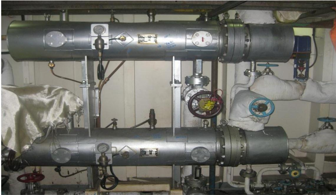
**Figure 11.8.1 – Typical fuel oil heaters**
