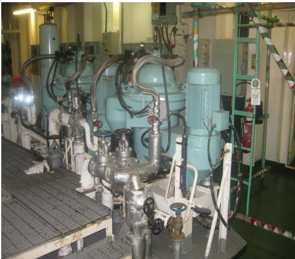
**Figure 11.7.2 – Typical purifier systems on-board**
