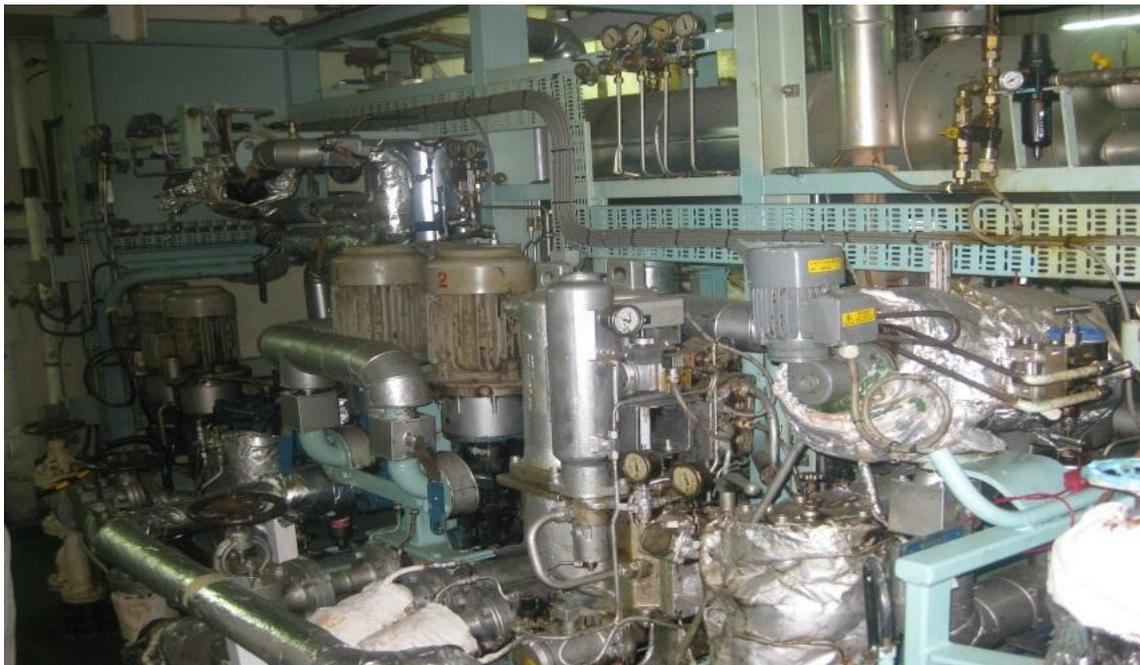
**Figure 11.8.2 – Viscosity controller and fine filter units**
